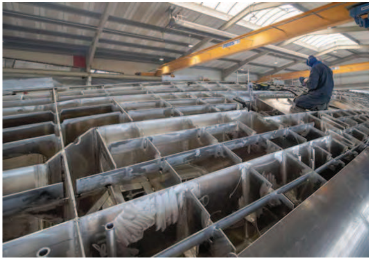
The ship was built entirely of aluminum using the proven net rib system
