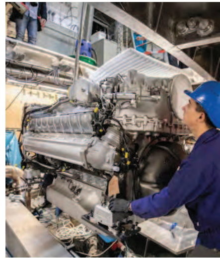
The engines are being installed
